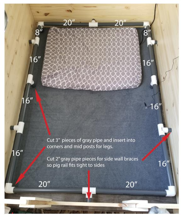
nect the 8" PVC piece and insert the other end of the 8" piece into the remaining opening in the back corner piece. Repeat these steps on the other 6 foot side. The fittings are tight so you can adjust the overall fit by tapping fittings with a hammer if the pig rail fits too tight and bows. See labeled photo below for visual of Pig Rail construction.
